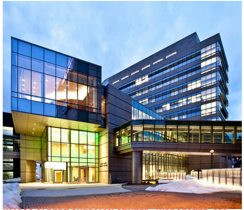
UMASS ALBERT SHERMAN CENTER- WORCESTER, MA
